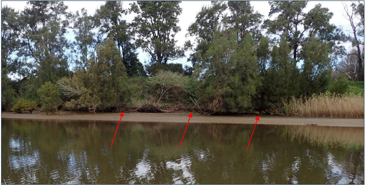
Figure 4: Representative photograph of bank scour along a bank section with an existing tidal bench. Note the partially detach root mat of the tree centre of picture and adjacent bank scour (identified by red arrows). Location is 550 m upstream of Terara Sands depot site. Flow is right to left.
