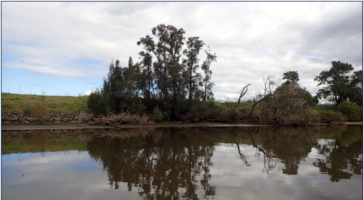
Figure 3: Representative photograph of episodic tree fall, likely associated with wind-generated wave action impacting the bank during the tidal cycle. Note the toe protection stone present along the bank in the left of the image and recruitment of mangroves upon the tidal bench. Location is 75 m upstream of Terara Sands depot site. Flow is right to left.
